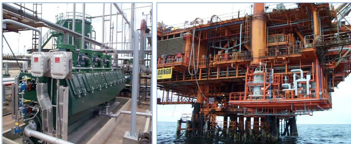
**Figure 2. (left) Four-stage mechanical IGF cell installed at a land-based oil facility and (right) a vertical IGF cell (gray vertical vessel near center) installed on an offshore fixed-platform.**
