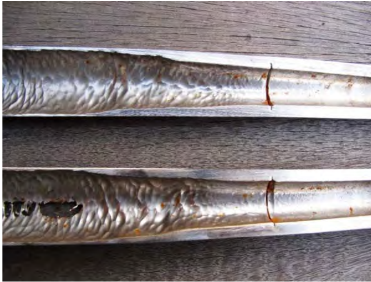
Figure 5. Erosion pattern marks on a 1.5" diameter desander showing premature failure in the cone section due to choked apex. Solids trajectory is from left to right. The cone section (left) shows severe wear while the apex (right) shows little or no erosion.
