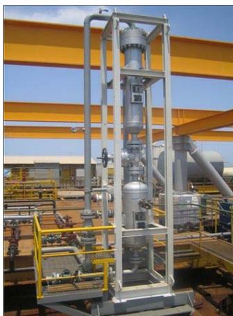
Figure 4 – Photograph of 900# wellhead desander system installed on shallow platform in Caspian Sea.
