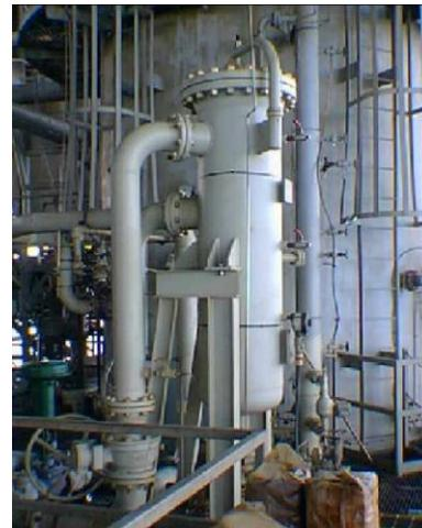
**Figure 3 – A 20,000 BPD desander for removing solids >10  $\mu$ m from the water stream after a production separator.**
