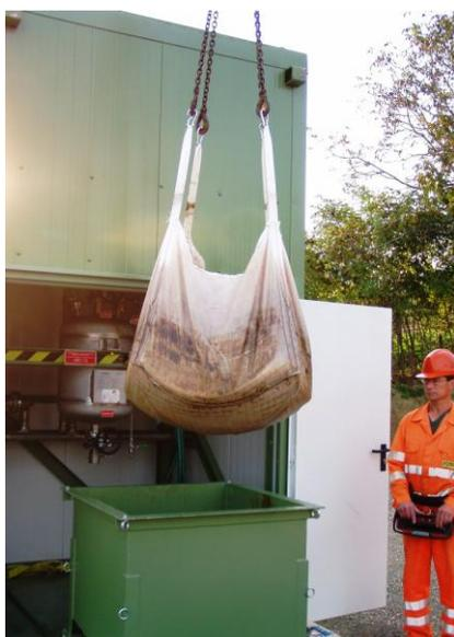
Figure 4 – Dewatered solids removal for dumping after separation from wellstream fluids with a desander.
