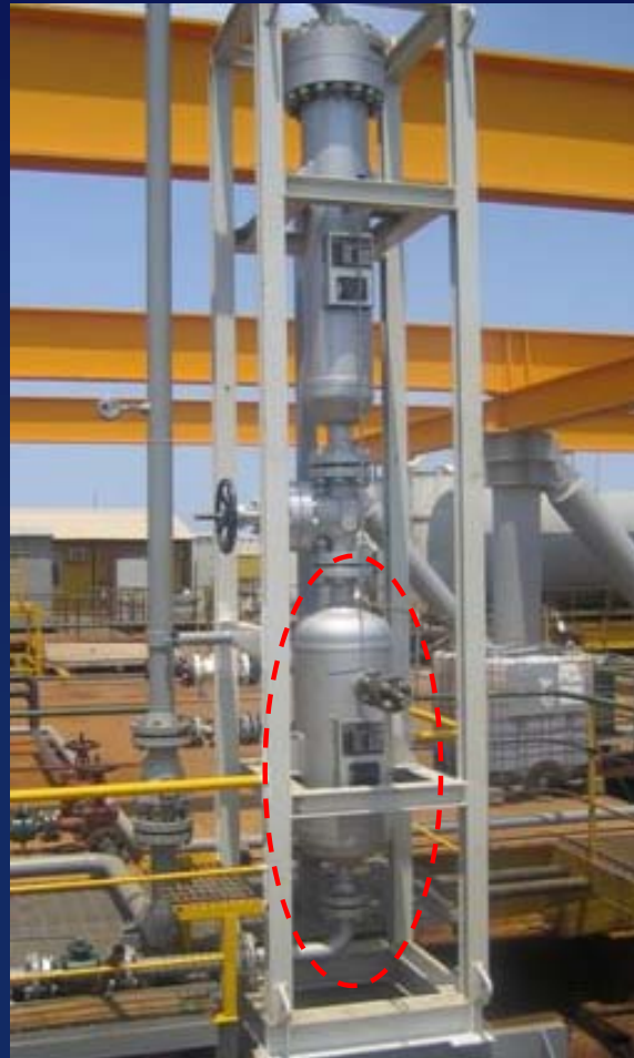
Wellstream Desander Acc. ASME 900#, 108 liter Turkmenistan 2011
