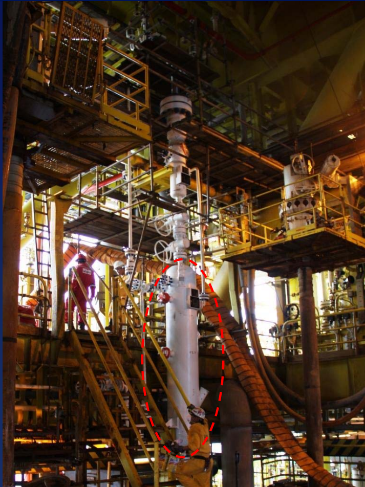
Wellhead Desander Acc. ASME 1500#, 600 liter Malaysia 2011
