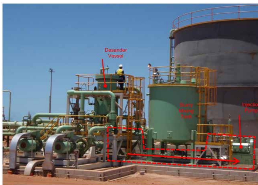
Figure 7—Transport of slurry from a produced water desander to an injection pump in an onshore Australian application.
