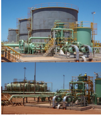
2007 Chevron Barrow Island Australia Pipe to Slurry Injection
