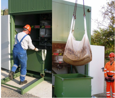
2005 R.A.G. GA Field Austria Dewatering Bag to Truck
